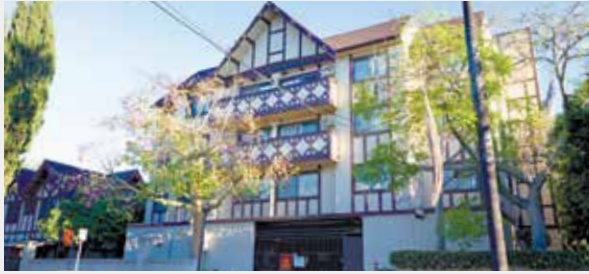
ANNENBERG HOUSE (ANH) 711 West 27th Street, Los Angeles, CA 90007
